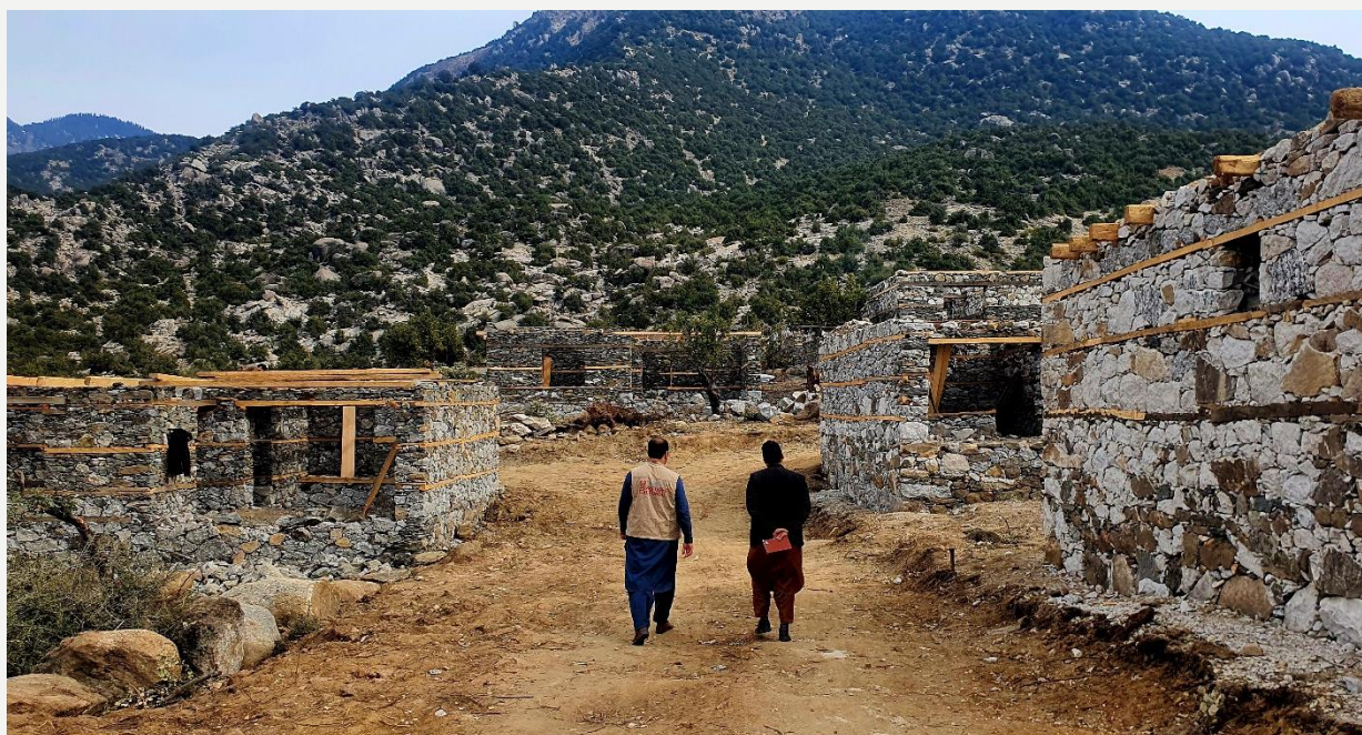
Photo 7. DRC Engineers monitor the construction works of Quba village.
