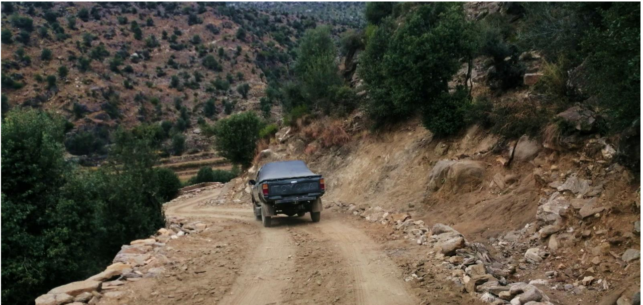
Photo 6. Ease of travel among local residents has significantly improved following the completion of the road network.
