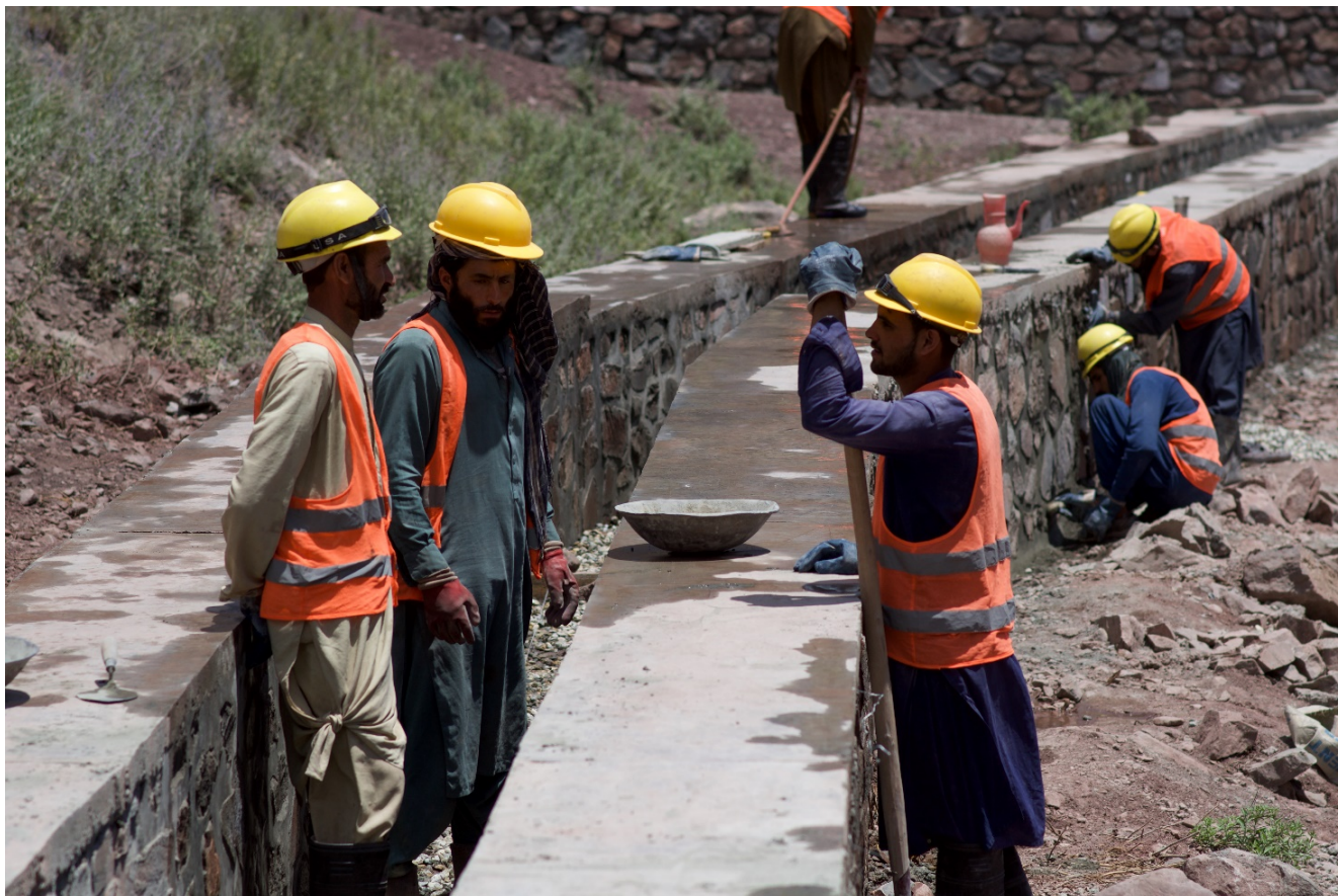
Figure 6: A group of men employed through a cash for work scheme work on the rehabilitation of the intake canal, July 2023
