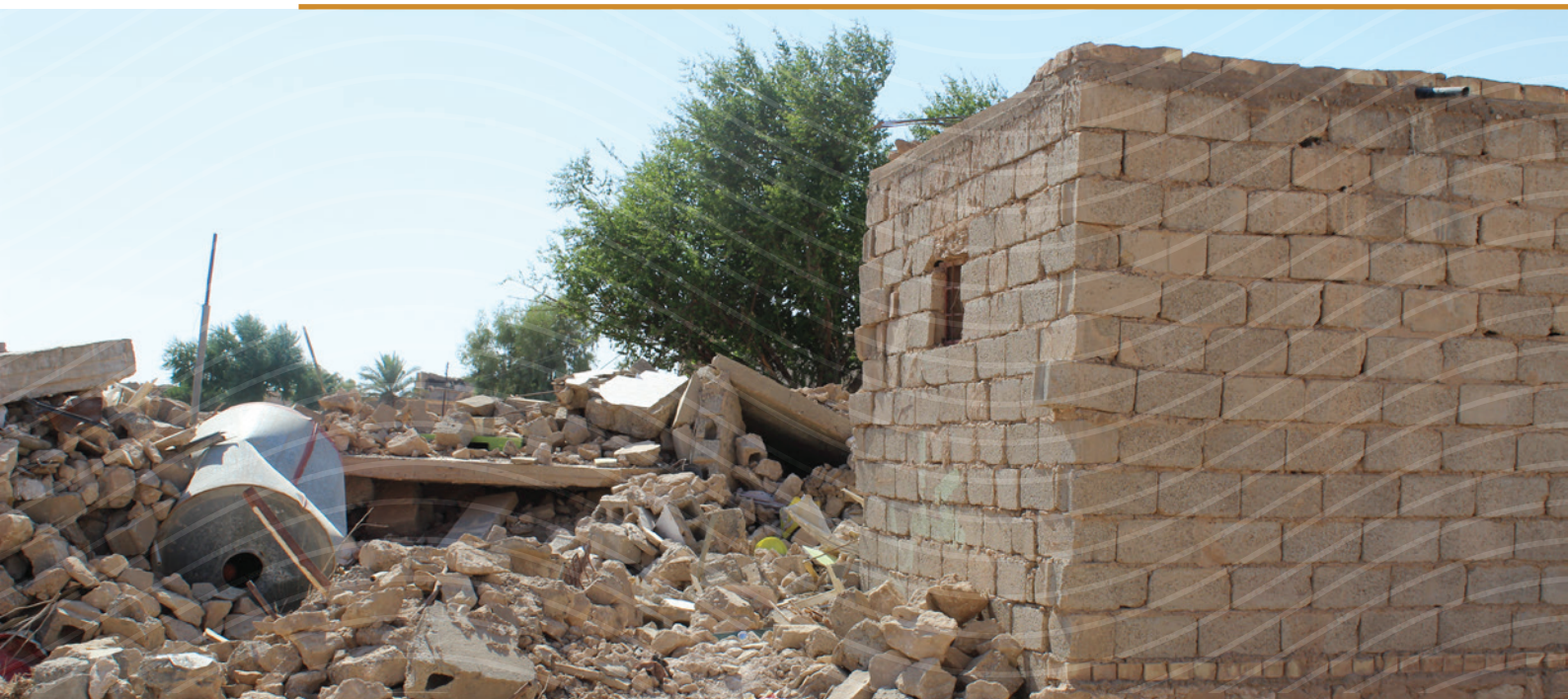
Damaged housing in Salah al-Din. Photo: Elysia Buchanan/DRC
