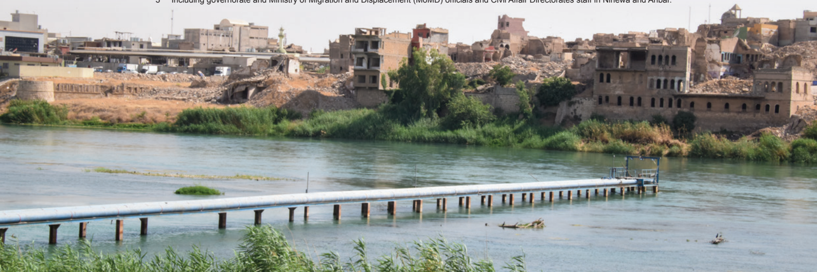
Buildings throughout the old city of Mosul remains destroyed years after large-scale conflict Photo: Ahmed Kaka/NRC
